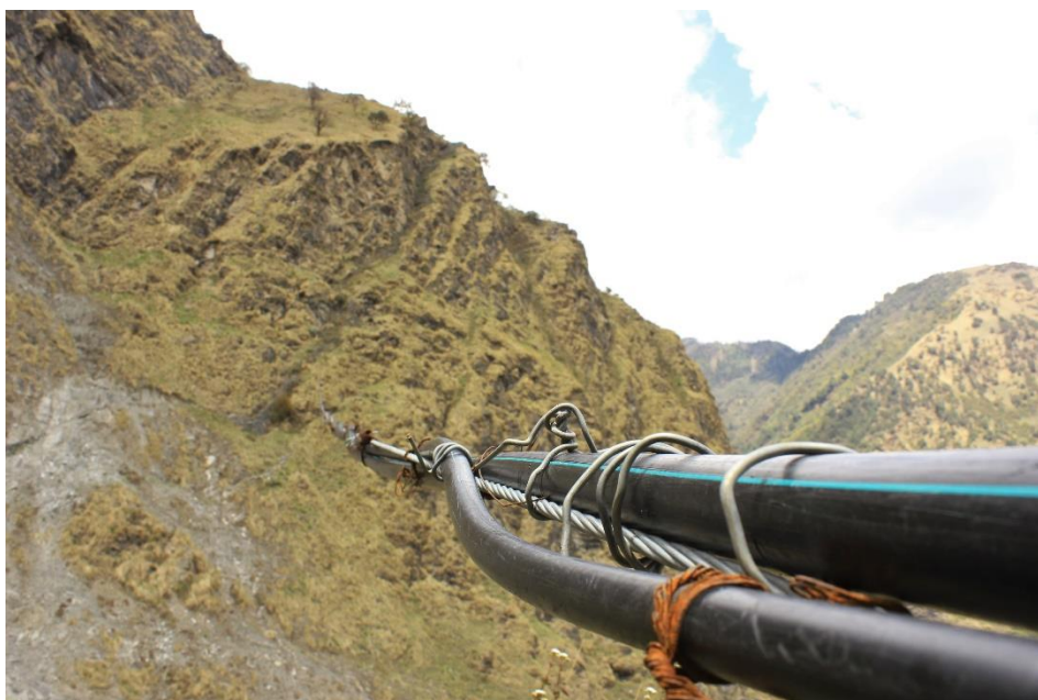
A 230-meter long suspended cable allows pipes to bring water from a water source over 5 kilometers away, across a deep gorge, into the village of Kupchet.
